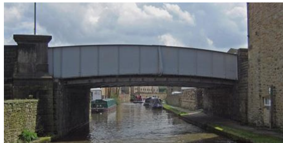
Bridge 179A – Pinder Bridge
