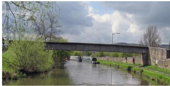
Bridge 179D – Footbridge
