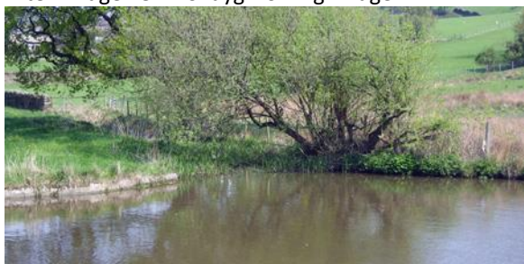
After Bridge 182A – Bradley Swing Bridge
