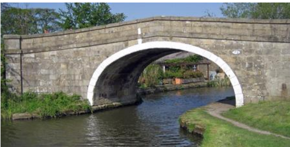
Bridge 172 – Ray Bridge W3W: soft.brain.grounding
