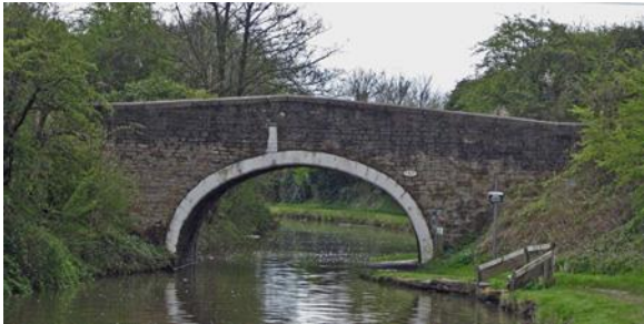
Bridge 180 – Horse Close Bridge
