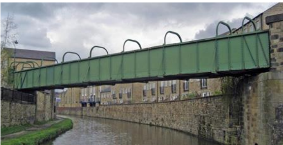
Bridge 179C – Tin Footbridge
