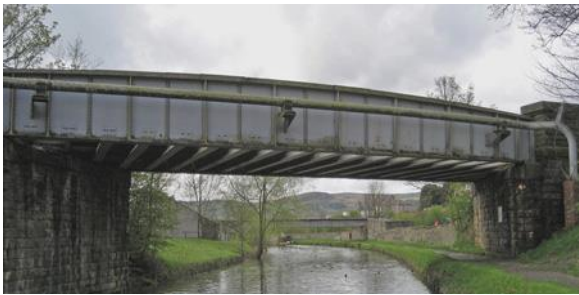
Bridge 179B – Dry Dock Mooring
