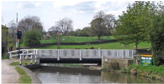
Bridge 187 – Warehouse Swing Bridge W3W: plodding.width.uncle
