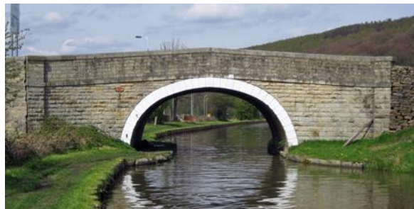
Bridge 183A – Farnhill Bridge
