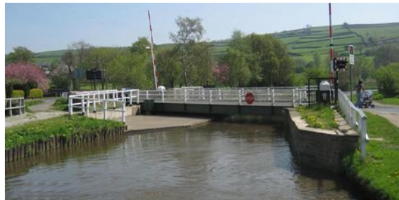
Bridge 182A - Bradley Swing Bridge W3W: fictional.emotional.tower
