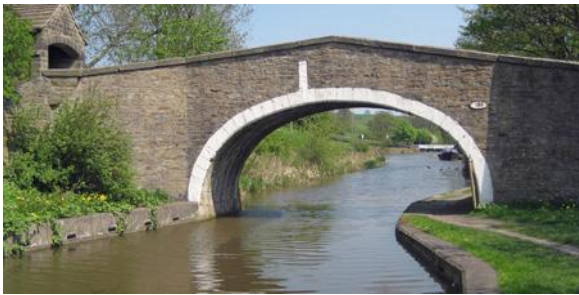
Bridge 186 – Parsons Bridge
