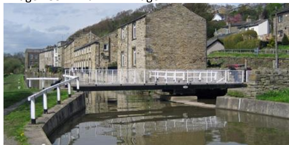
Bridge 185 – Redmans Swing Bridge
