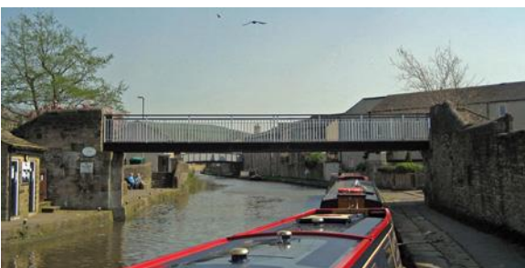
Bridge 179 – Gallows Footbridge
