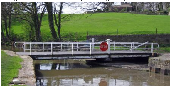
Bridge 184 – Milking Hill Swing Bridge
