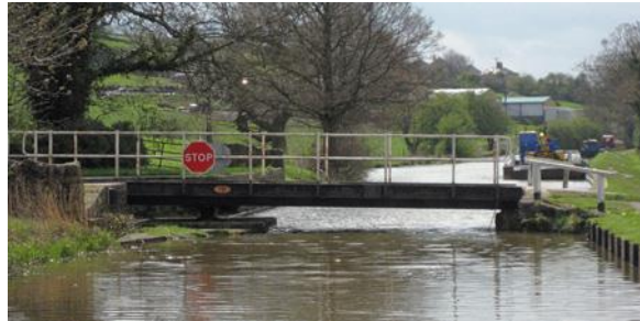
Bridge 181 – Snaygill Swing Bridge W3W: seasonal.spouting.broke
