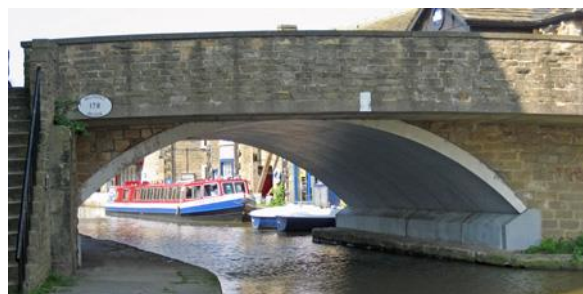
Bridge 178 – Belmont Bridge W3W: rejoin.skies.prop
