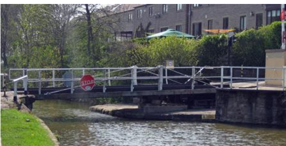
Bridge 177 – Brewery Swing Bridge
