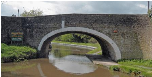
Bridge 182 – Snaygill Stone Bridge
