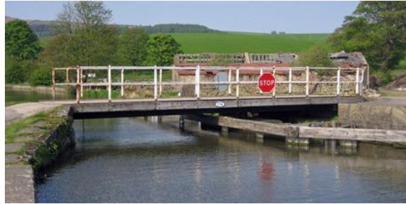
Bridge 174 – Thorlby Swing Bridge
