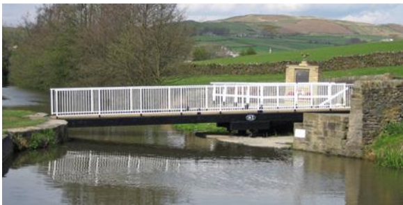
Bridge 183 – Hamblethorpe Swing Bridge
