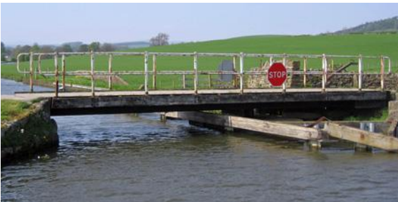
Bridge 173 – Highgate Swing Bridge W3W: clown.wager.elevator
